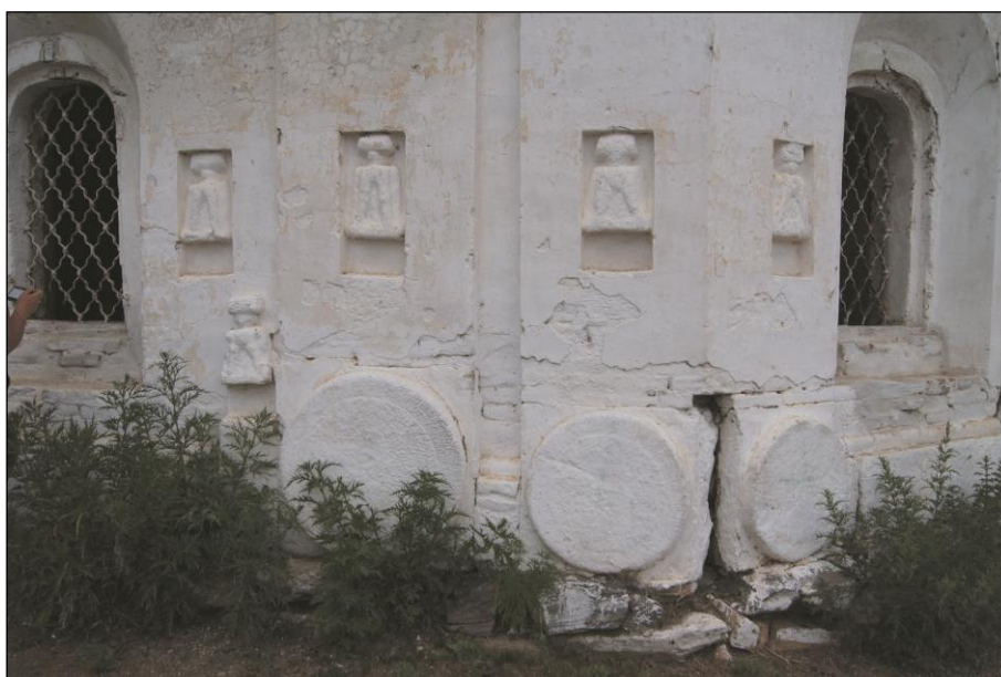
Fig. 7. Pilar foundation and stone dragons from palace in Kondui Orthodox Church
